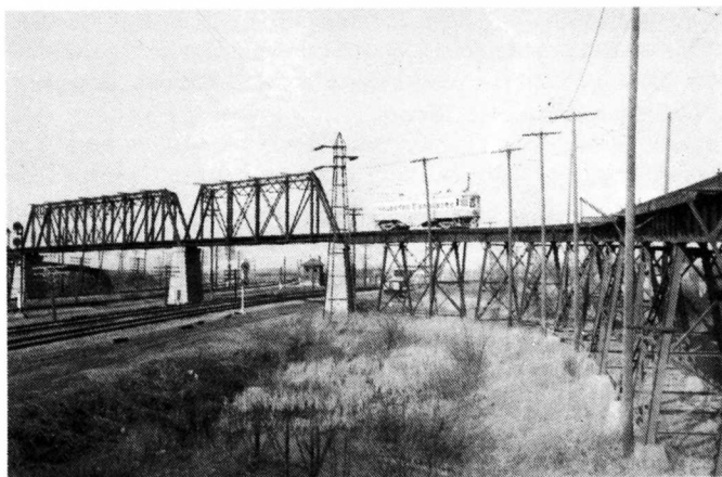
An Illinois Terminal interurban car southbound from Alton crosses over the interlocking plant at Lenox on April 13, 1952. Courtesy of the TRRA Historical & Technical Society.
