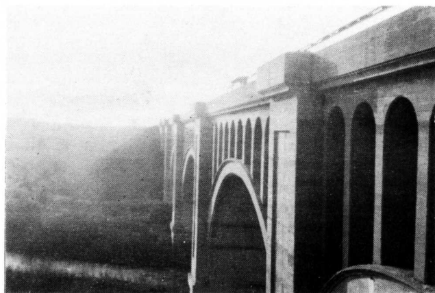
The viaduct over the Okaw River north of Findlay as it appeared in 1936 before the impoundment of Lake Shelbyville. Barriger Collection, Mercantile Library.
